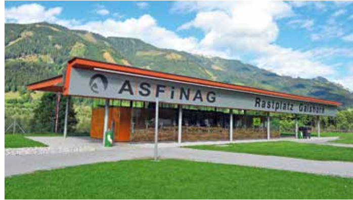
Figure 10: ASFINAG service area
